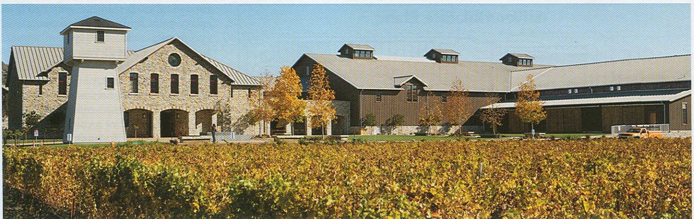
The raised 3.7 acre building site hovers at the same height as the top of the adjacent vineyard. From left to right: Hospitality Building (with iconic water tower in front and obscured Administration Building behind), Fermentation, and Barrel Storage.
