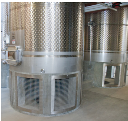
CO 2 sinks/enters the below-ground cavity under tanks (left), and an exhaust fan outside the building vents the CO 2 coming out through ducts (right) into the vineyard in front of the winery.
