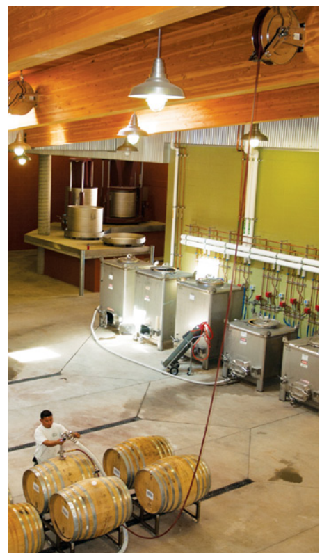
Easy removal of barrels from storage cell (left) to indoor barrel working area (left, background). Two reels drop nitrogen hoses from the ceiling (right) to provide nitrogen for a Racketeer debarreling wand, keeping the floor free of hose congestion for unencumbered activity.
